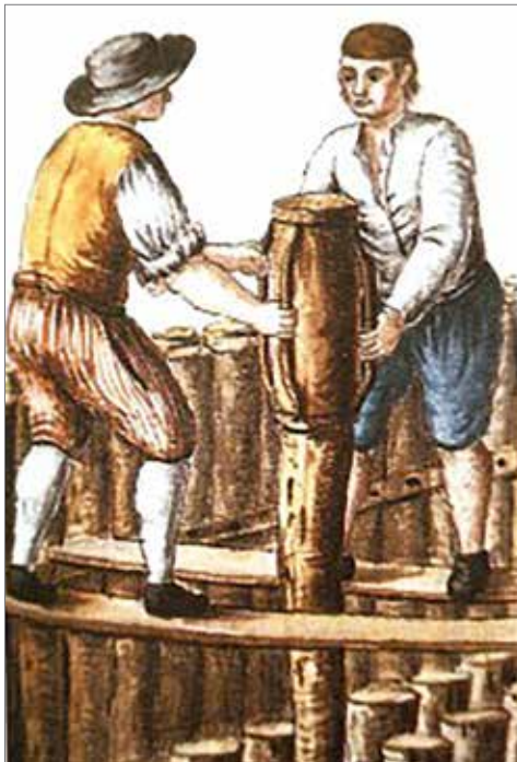
Figure 6. Eighteenth century pile drivers working on the foundations for a Venetian church.
