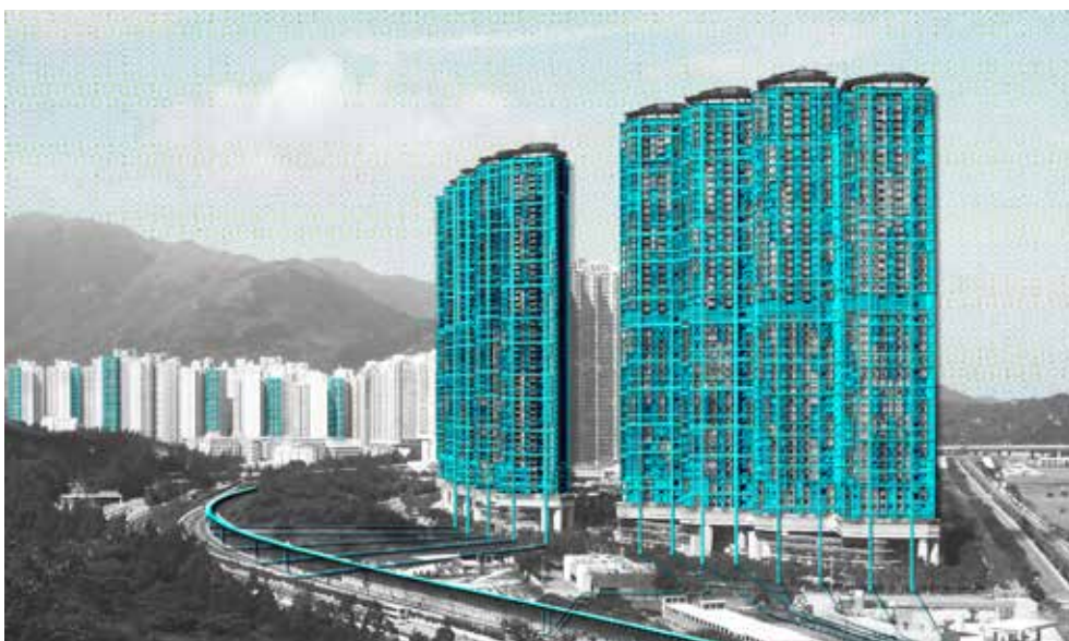
Figure 2. Wastewater collection and vertical water treatment systems are layered onto the facades of residential towers to take advantage of gravity-driven purification systems.
