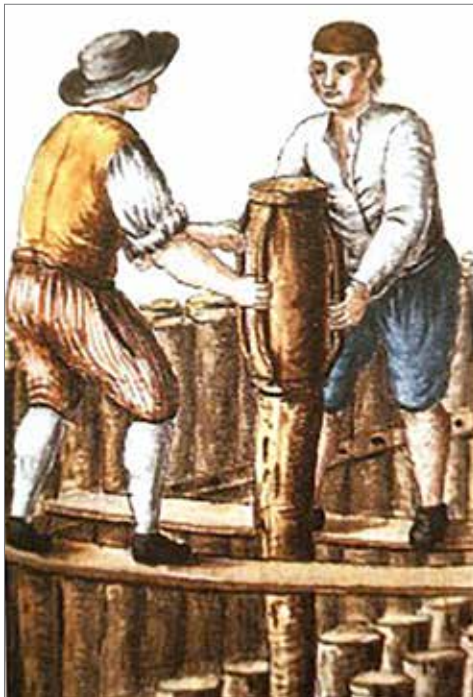
Figure 6. Eighteenth century pile drivers working on the foundations for a Venetian church.
